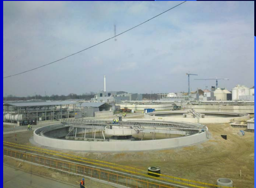
WWTP Czajka in Warsaw
